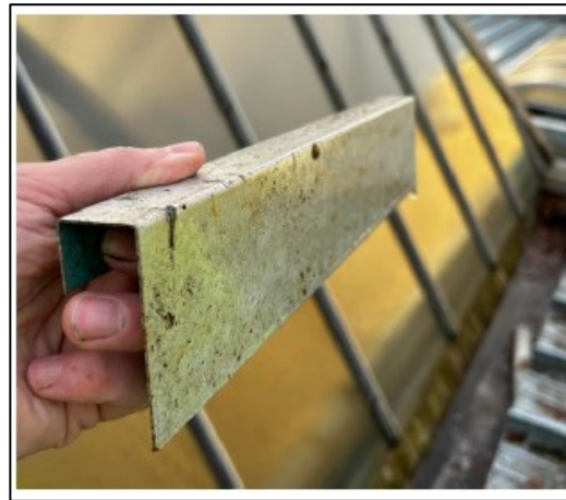
Figure 3: Loose ridge drip trim.
