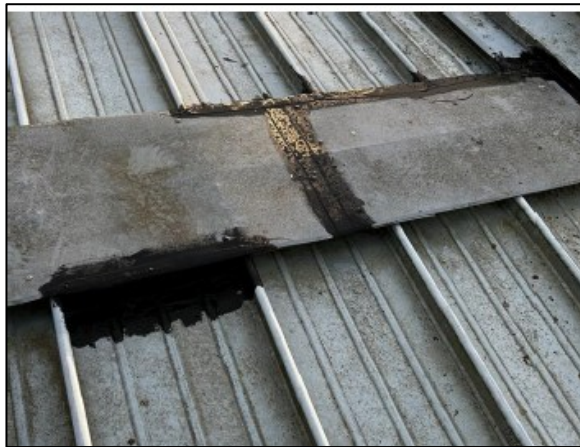
Figure 2: Existing ridge detail with signs of past repair.
