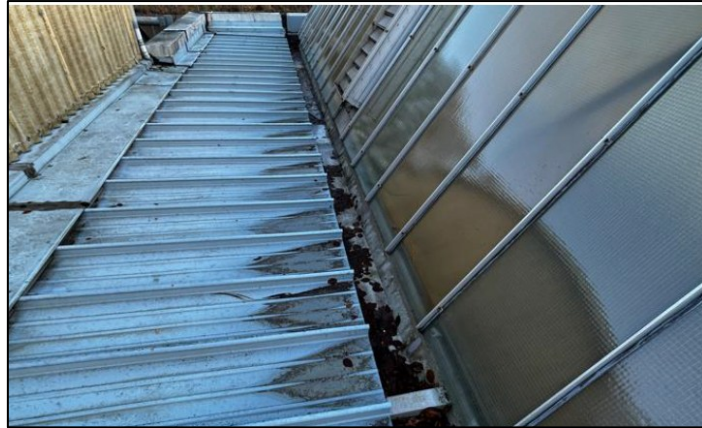
Figure 1: Damaged sheets w/ water pooling
