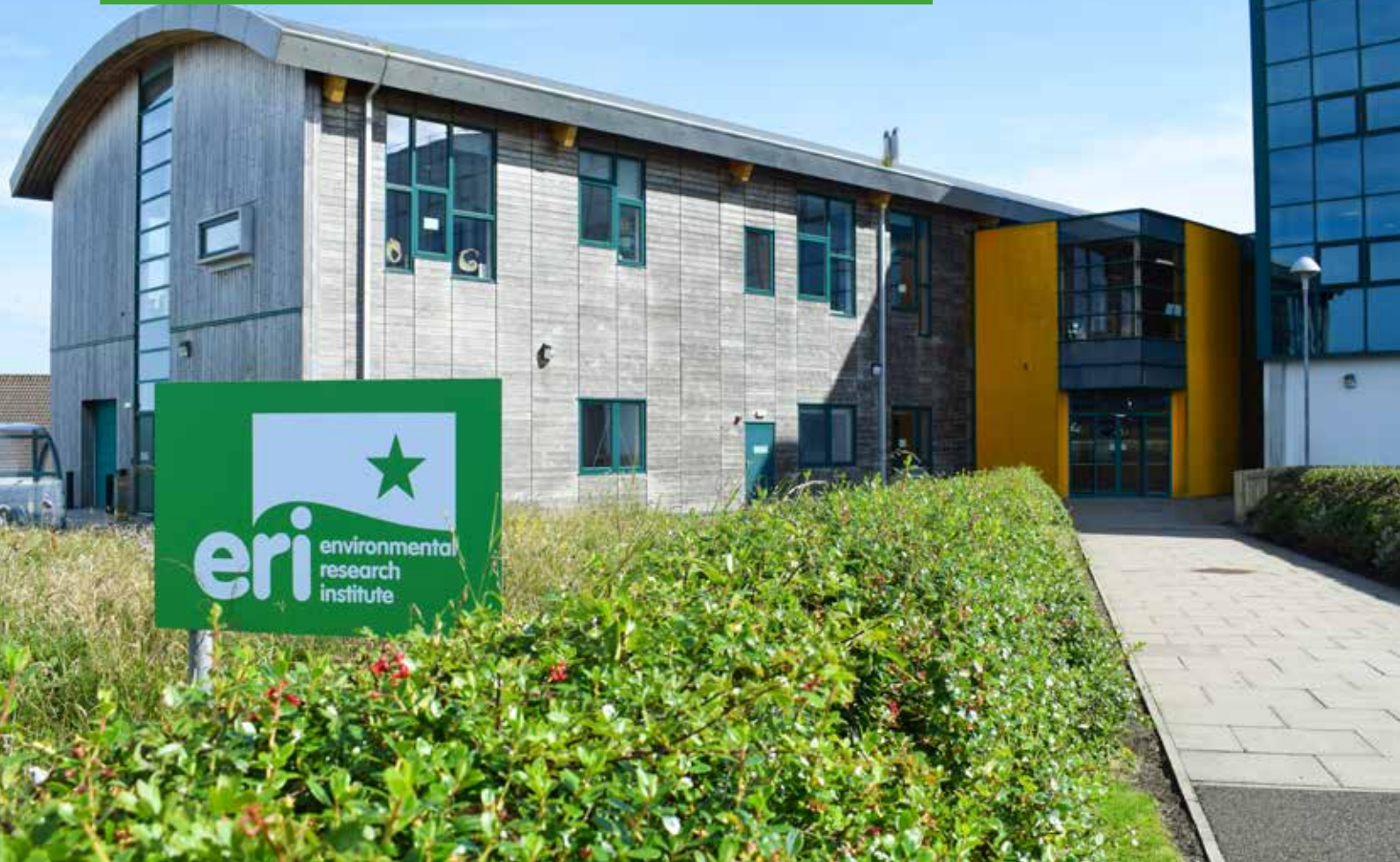
ERI - Centre for Energy and the Environment, Ormlie Road, Thurso
